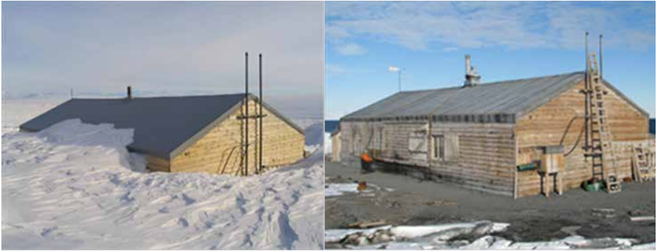
FIGURE 2 At Captain Scott's historic hut and the other historic huts on Ross Island, Antarctica, an annual monitoring programme of temperature, relative humidity, snow, and building movement is in place following a major programme of conservation of the buildings and artefact collections. Photograph (nzaht.org)
