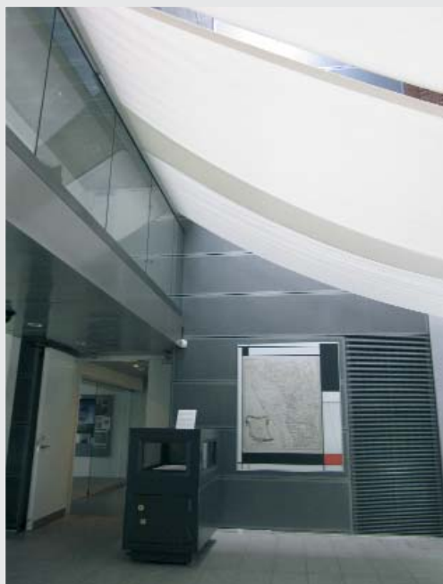
12 Awnings lowering the illumination from the skylights.
