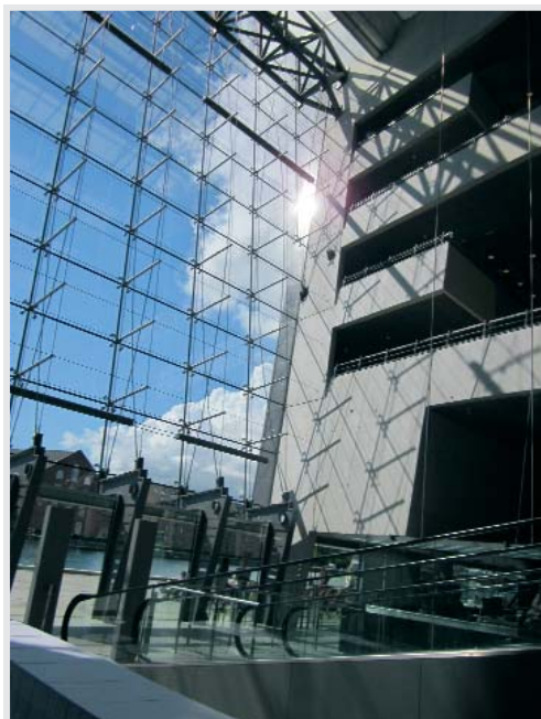
5 Reflection of sunlight from the shiny stone facade results in lux levels of more than 10,000 in a preinstalled showcase (not visible but behind the back of the photographer) for a short while during the daytime.
